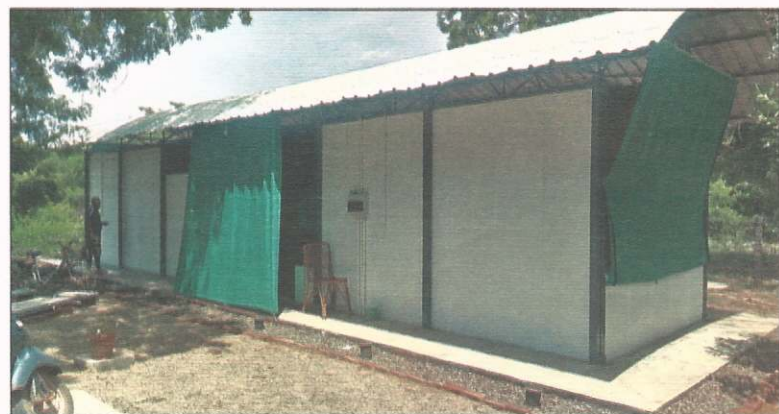
Low-cost house in Pony Farm community. The walls are styrofoam-cement sandwich panels
