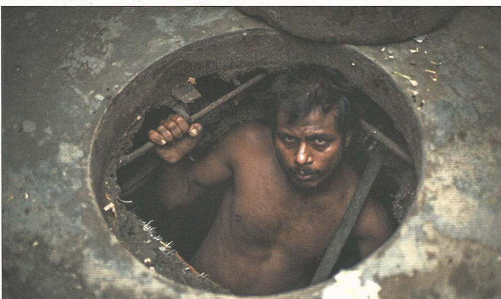
A conservancy worker descends a manhole to clean out a blocked drain
