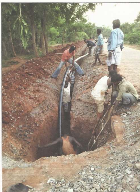
Laying HDPE pipes along the Crown road
