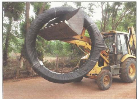
Transporting HDPE water pipes
