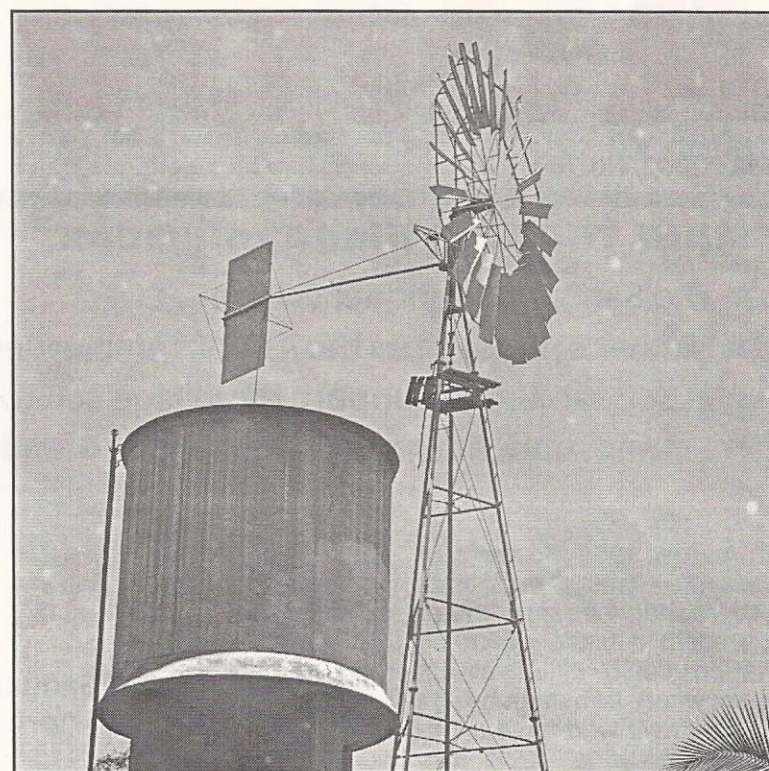
Made in Auroville: windmill and ferro-cement water tank
