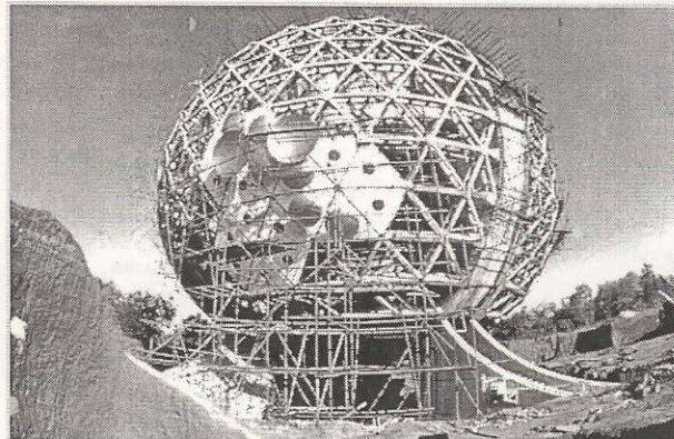
This fish-eye view of Matrimandir shows the first try-outs to fill the space-frame with ferrocement triangles, and the first samples of the discs.
