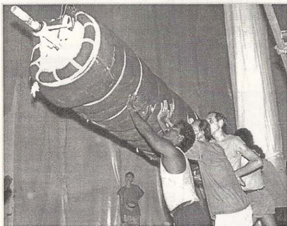
Lifting the pillars to their places in the chamber. Right: The chamber with pillars in place but still without the crystal
