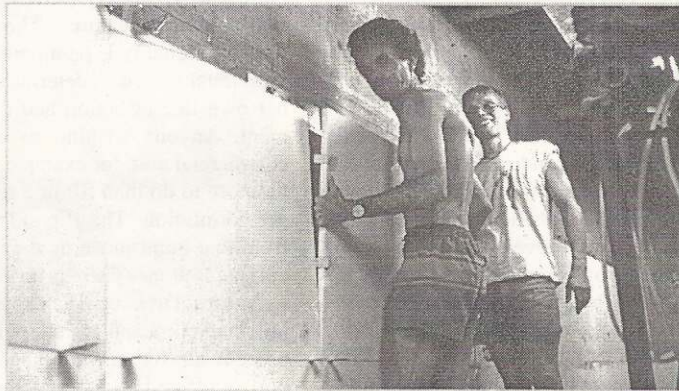
Top: Installing the marble in the chamber.
