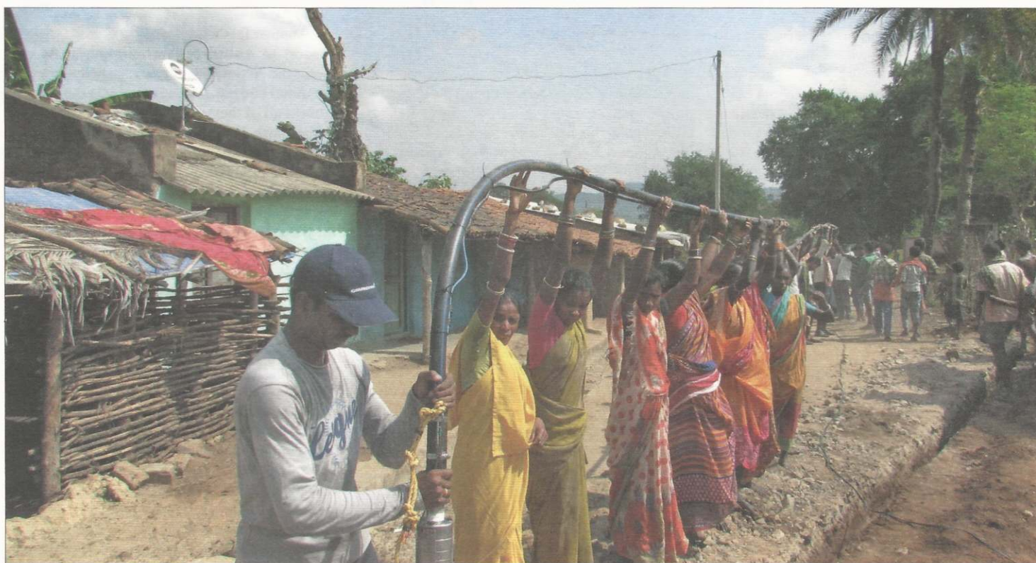
Installing a solar pumping system in Gobada village, Orissa
