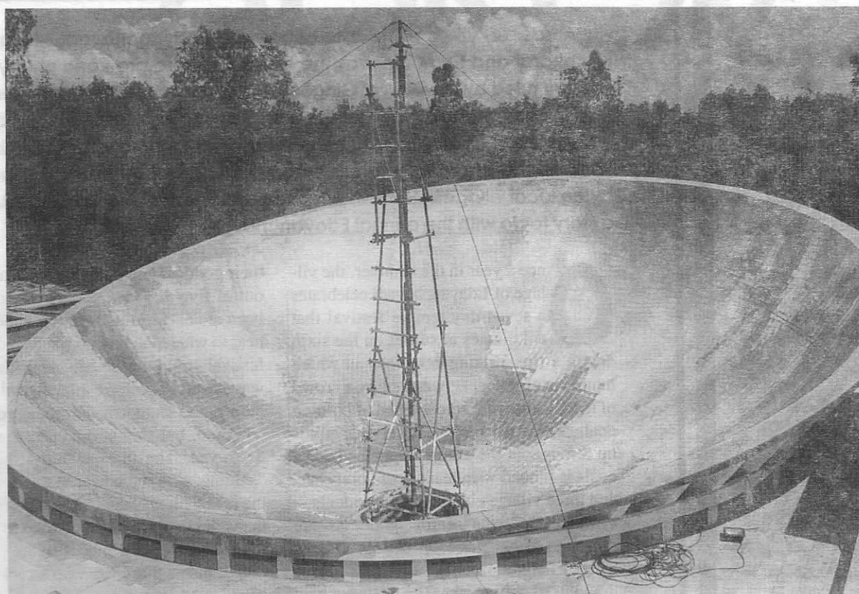
The fixing of the glass mirrors to the solar bowl at the Cuisine Solaire Pour Tous, or Solar Kitchen, is now complete. The bowl is expected to be operational in August.
