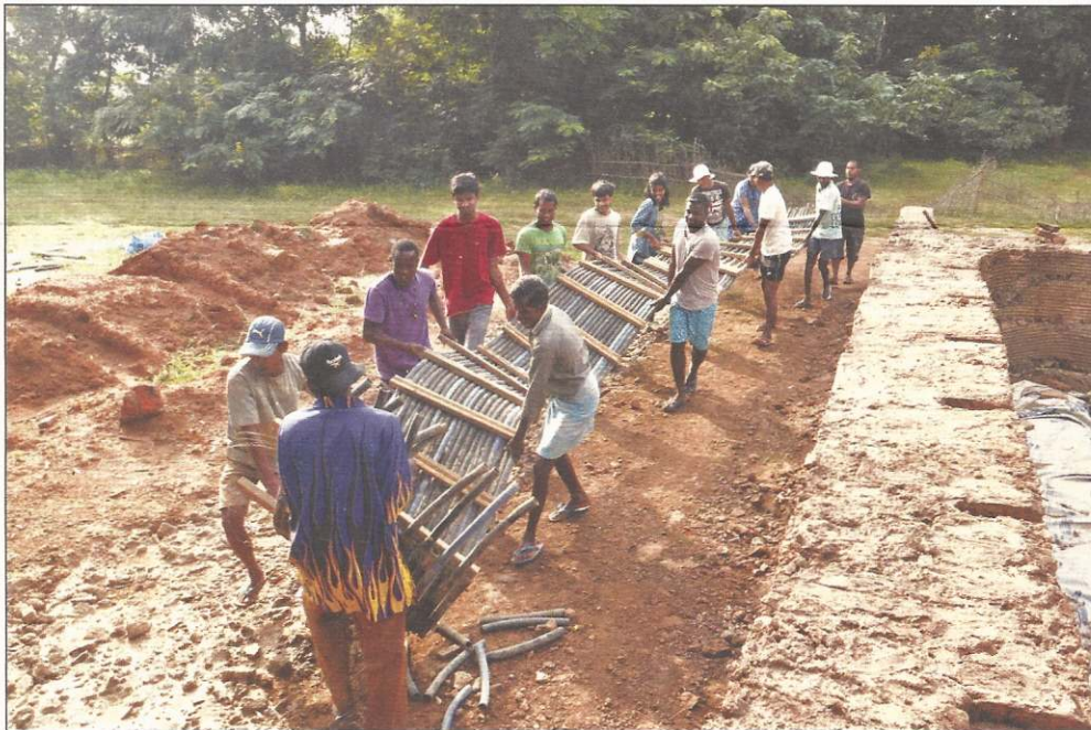
Moving the shuttering made from discarded petrol pump pipes into position for building the walls
