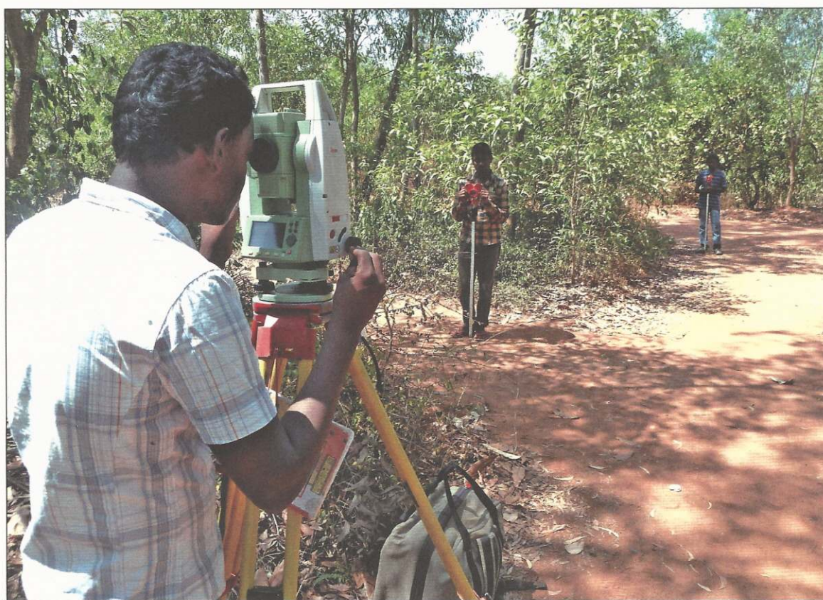
Surveying the new Transition radial road
