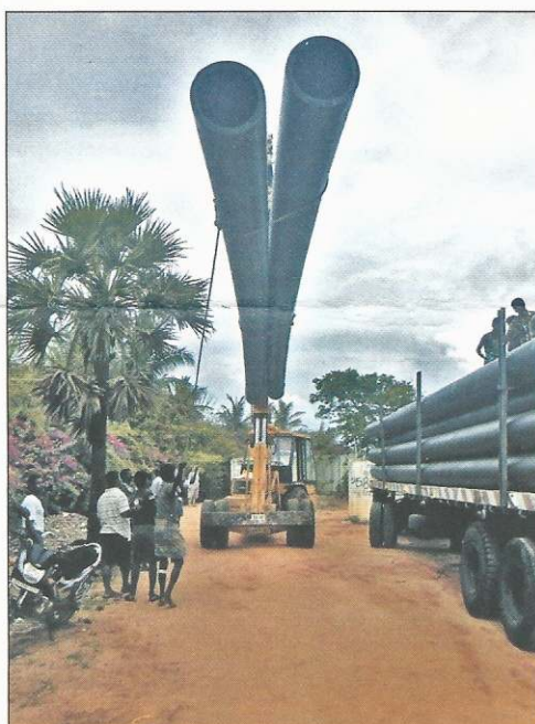
Unloading pipes to transport water from the site of the desalination plant to Auroville
