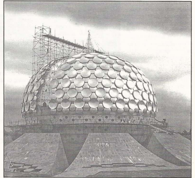
Monsoon clouds gather behind the Matrimandir. The scaffolding necessary to remove the crane is still in place. The last remnant of the crane, the triangular structure on top, is the last piece to be removed.
