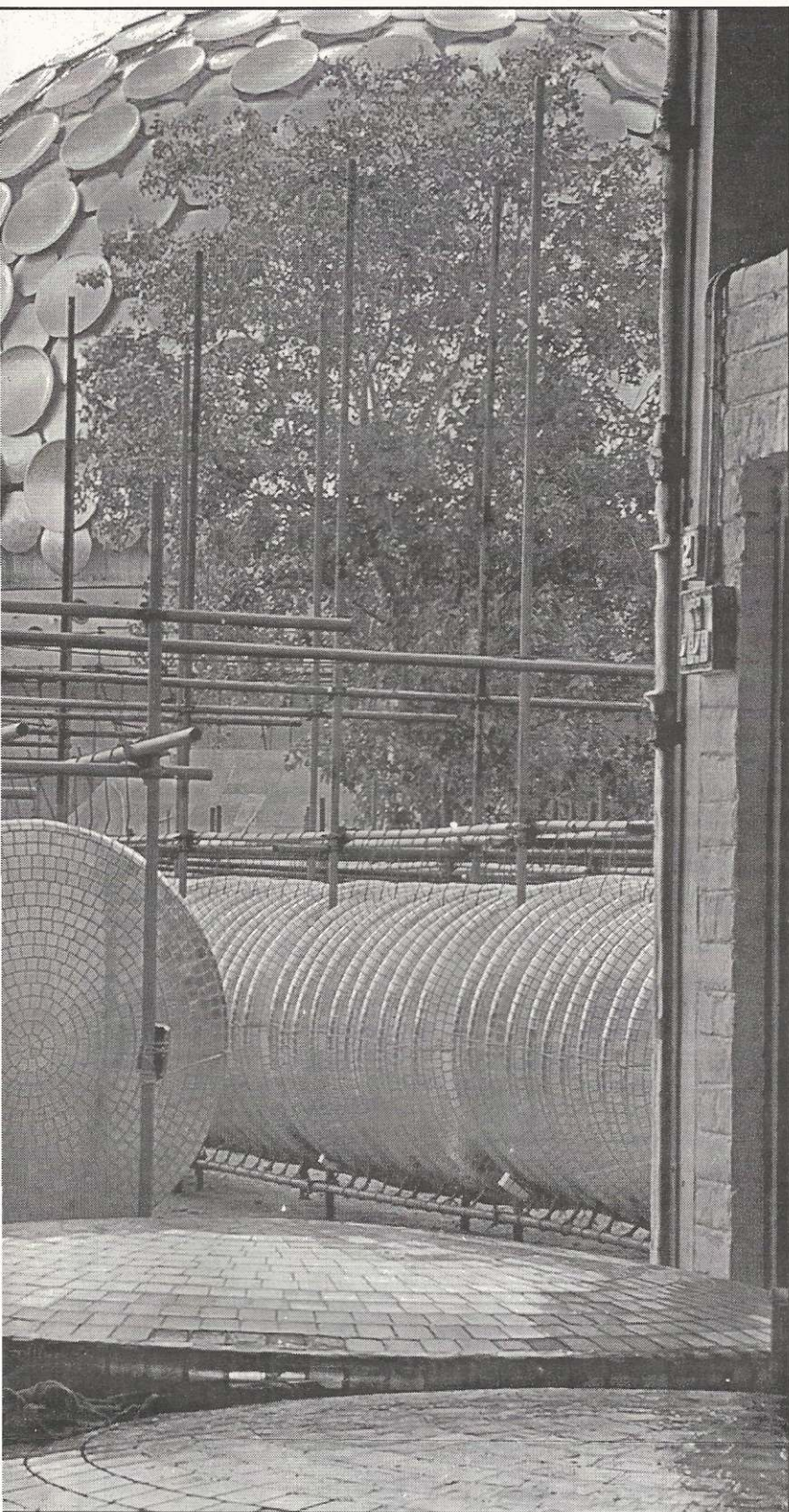
View on the Matrimandir from the discs workshop. Less than 50 discs still need to be clad with the golden glass tiles. The fixing of the discs on the Matrimandir can be finished by June 2002.
