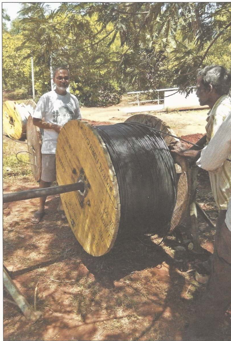
Chandresh supervising the laying of the optical fibre cable
