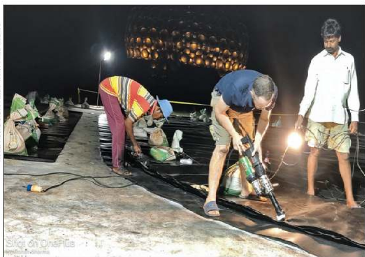
HDPE welding was done at night
