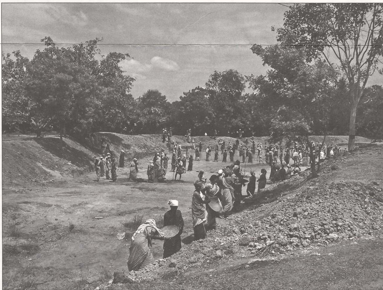
Desilting an Edaiyanchavadi tank.
