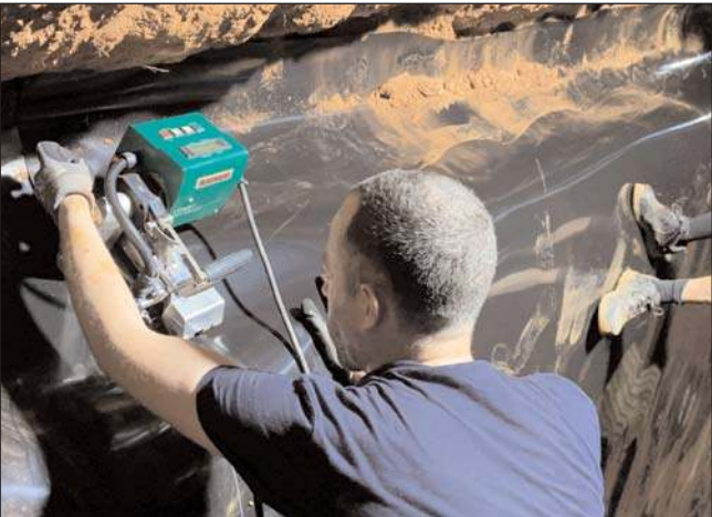
Welding the two mm thick HDPE sheets
