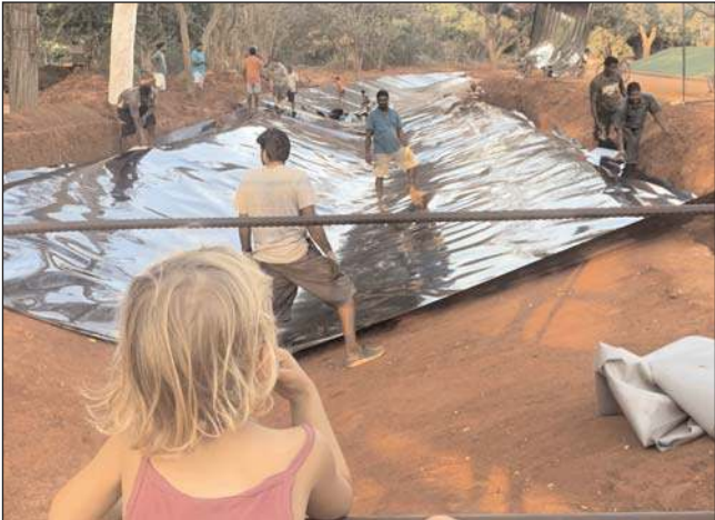
Installing the waterproofing liner
