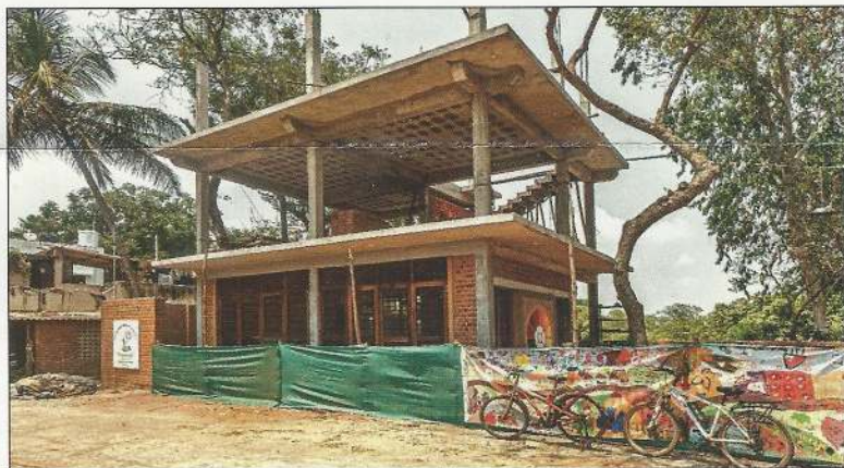
The new building under construction
