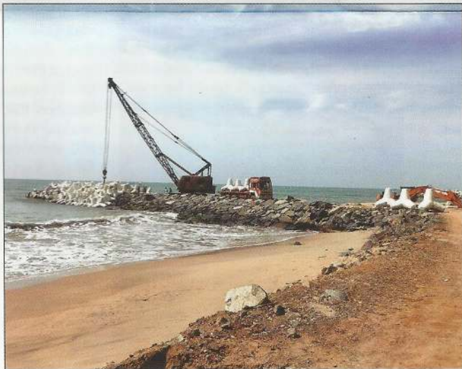
Building a groyne
