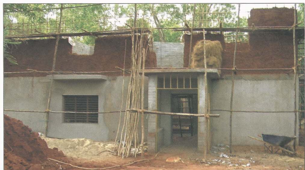
The house under construction: mud mixed with coir is applied to the bamboo; the walls are then cement-plastered
