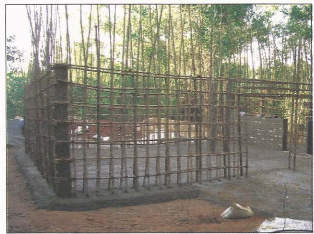
The bamboo grids for the walls stick out from the concreted floor
