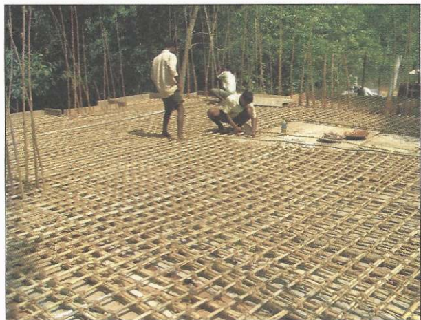
The bamboo grid for the first floor
