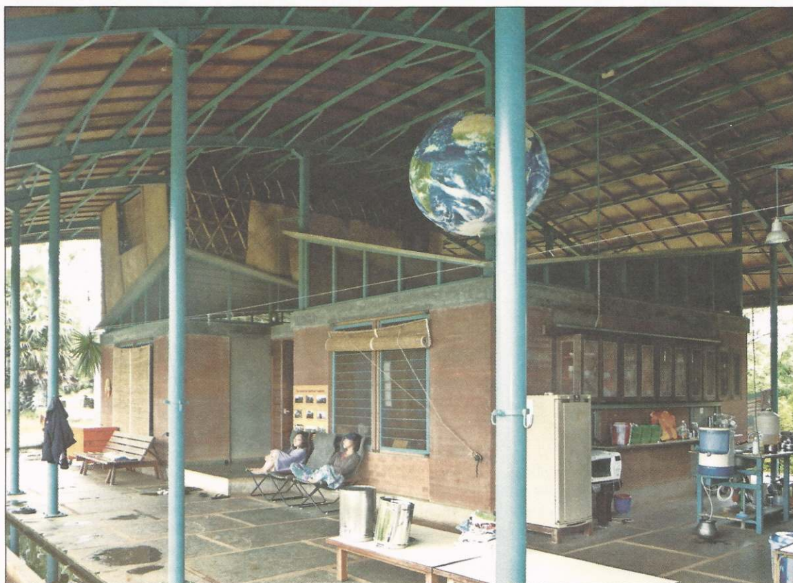
The 'super roof', a steel structure covered in wood, protects the inner dorm rooms, bathrooms and office
