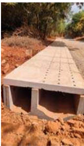
Ducts along an unfinished stretch of the Crown Road. All holes will now be closed.
