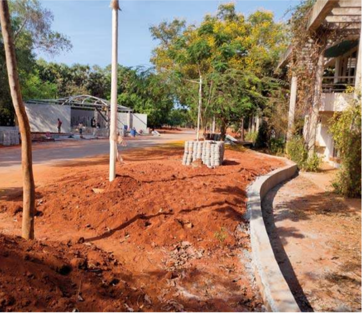
The Crown Road nearby Kalpana community. A retaining wall is being built to prevent earth from the roadside flushing into Kalpana.
