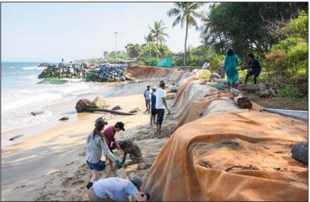
Protecting the coast with leftover cloth from the Matrimandir Lake construction
