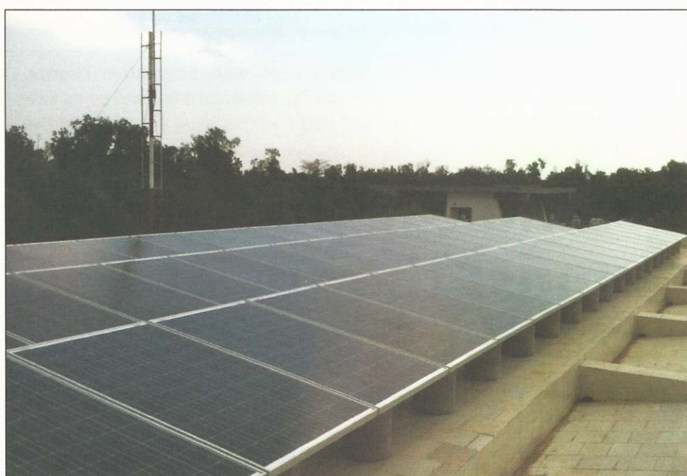
The 15 kW grid-connected solar photovoltaic plant on the roof of the Auroville Foundation building
