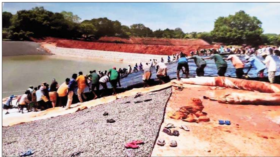
Placing the first underwater cushion for storing drinking water in the lake
