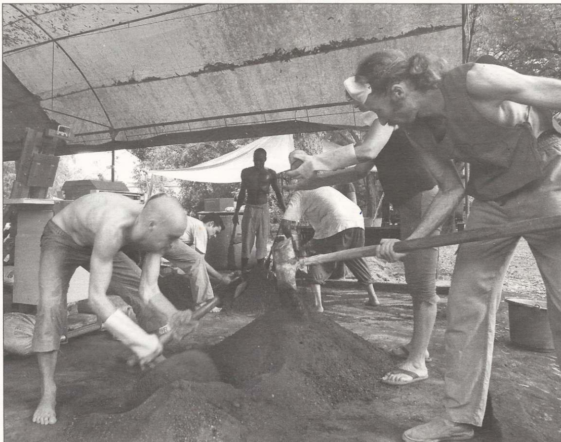
Newcomers and Aurovilians preparing mud bricks for house construction at the Auroville Earth Institute
