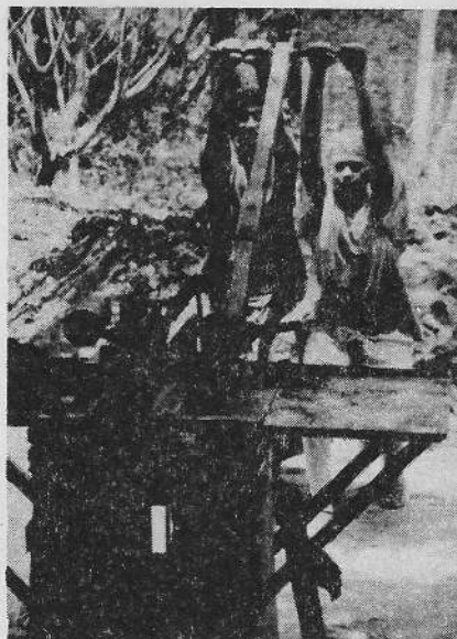
Compressing stabilized earth blocks
