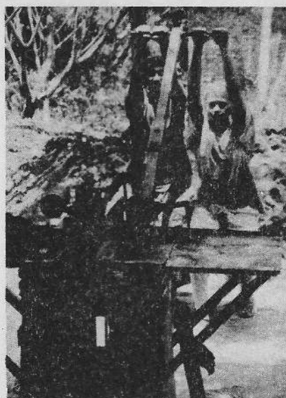
Compressing stabilized earth blocks
