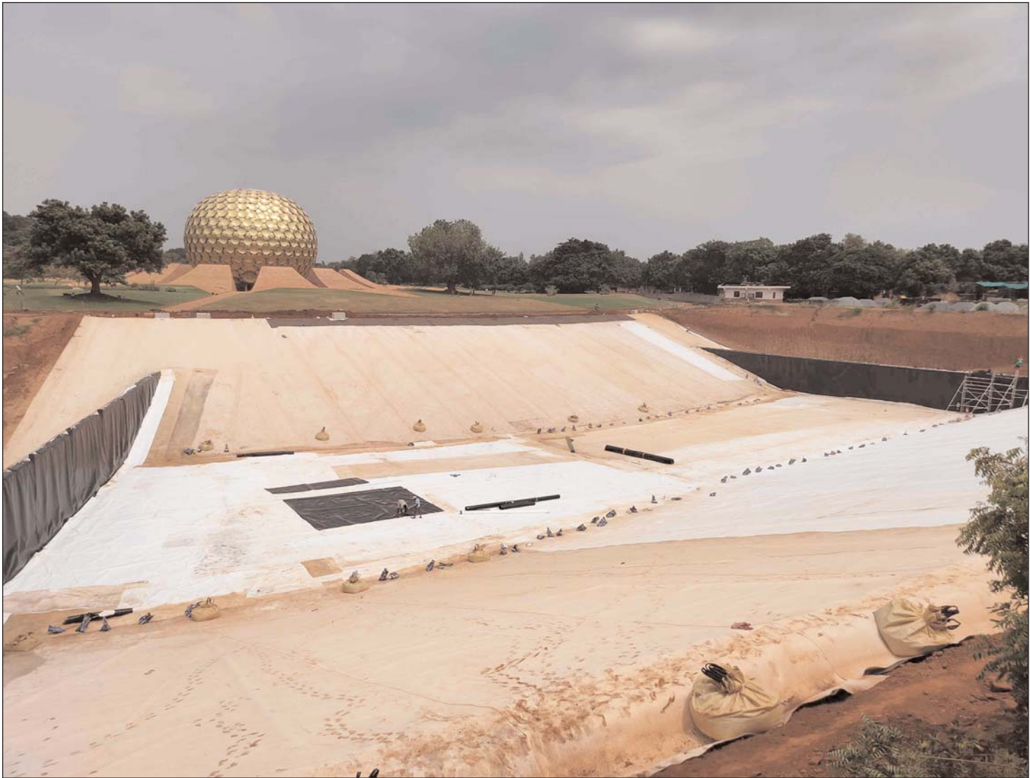
The almost completed Matrimandir test lake. Small granite chips will cover the white geotextile. The walls are clad with hdpe liner.
