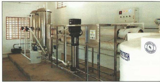
The reverse-osmosis desalination plant at the Quiet Healing Centre
