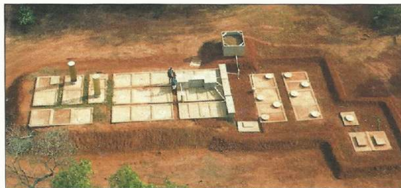
The centralized waste water collection system in the Residential Zone
