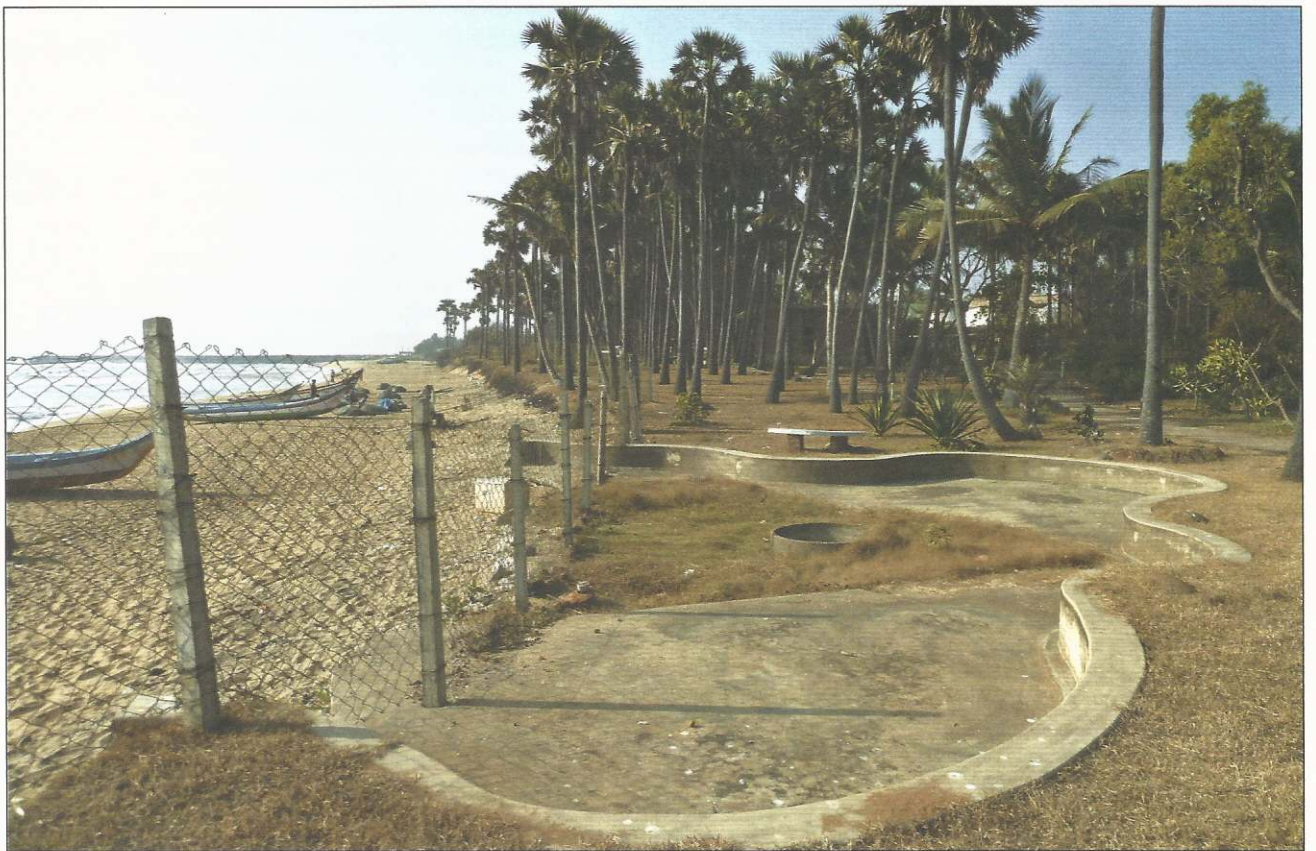
The erosion at Quiet Healing Centre has entered the compound, destroying an ornamental pond. The beach has returned temporarily, but erosion will resume within two months
