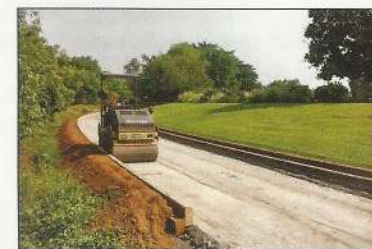
130 metres oval road being prepared for its surface cladding of granite cobble stones
