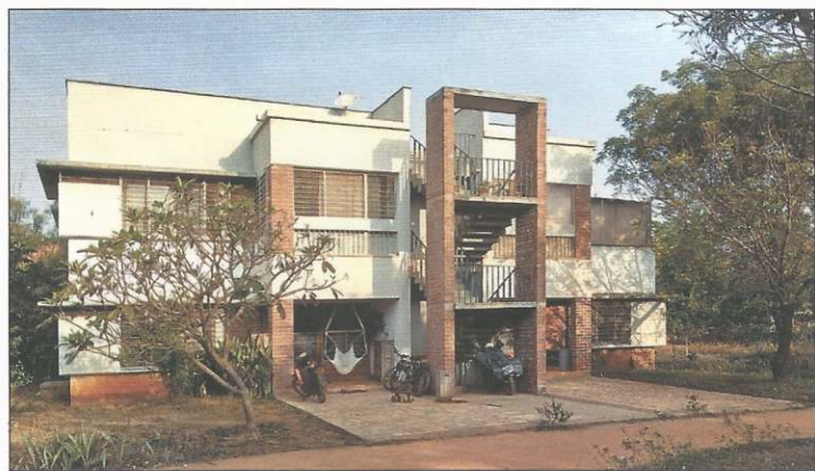
Apartments in Maitreye I. The roofs are leaking
