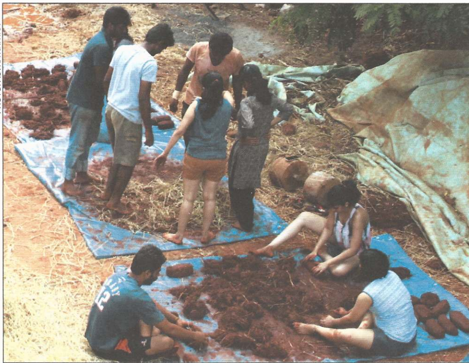
Preparing the cob mixture
