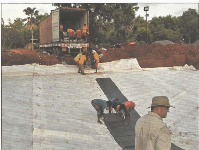
Laying compacted clay slabs on a geotextile under-layer in one of the six mini test ponds at Matrimandir
