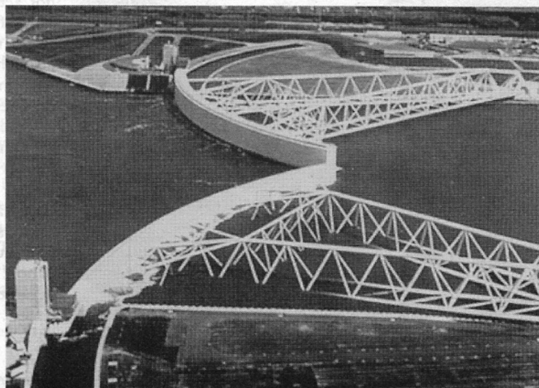
New storm-surge barrier in the New Waterway near Europoort, consisting of two enormous hinged gates spanning a width of 360 m.
