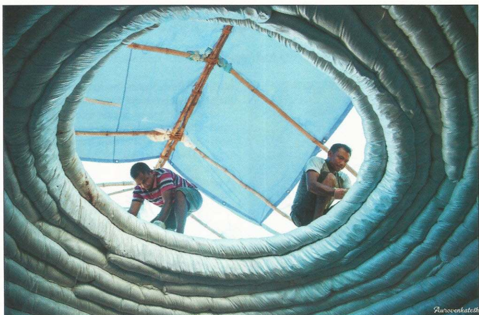
The earth bag house in the making
