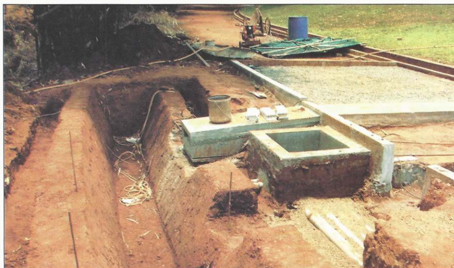
A trial sample of the open storm water collection channel being created at the edge of the oval road in April
