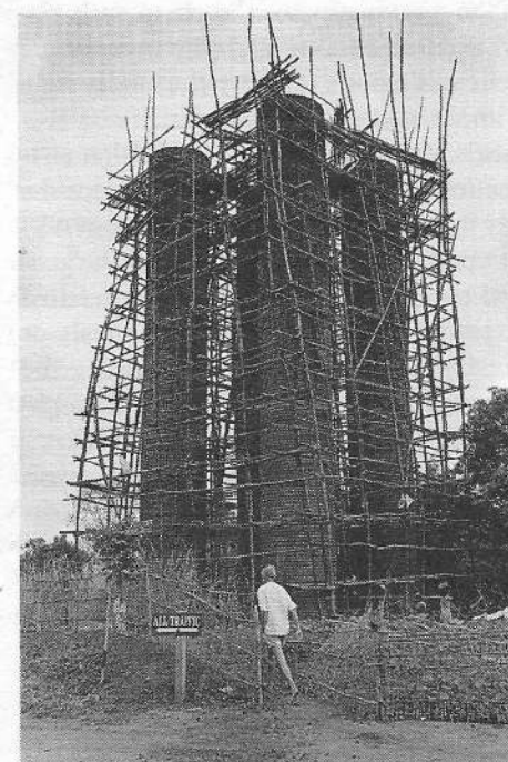
Towering water tanks under construction between Surrender and Arati. Architect: Helmut. These tanks are innovative in the sense that they will link wells of the various communities in the first sector of the RZ and provide water to all.
