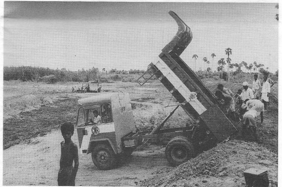
Water Harvest: Repairing the bund of a village catchment tank
