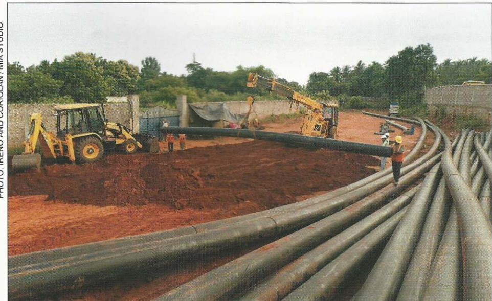
Butt-welded HDPE pipes at 'Guna's school'
